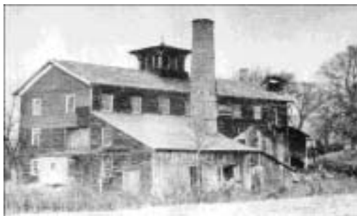
Known today as the "Old Mill," this 1858 structure actually replaced the original two-story building after it was seriously damaged by fire. The different tone of the upper and lower clapboards in this old picture may demarcate the line of the new topside construction. In its heyday, the third floor, Baker's Hall, was the site of many area dances and shows.
